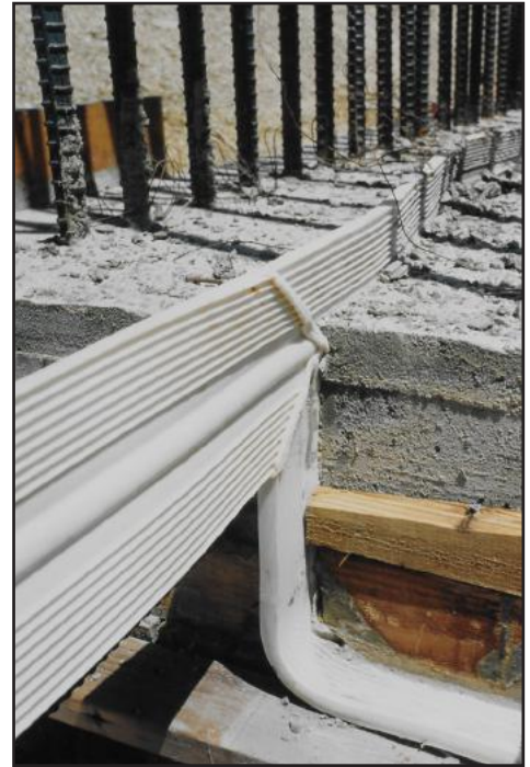
PVC978 (with eyelets: EYPVC978) 9" Tear Web Waterstop 125 ft Head of H 2 O • 50 lft/roll • 1.2 lbs/lft
